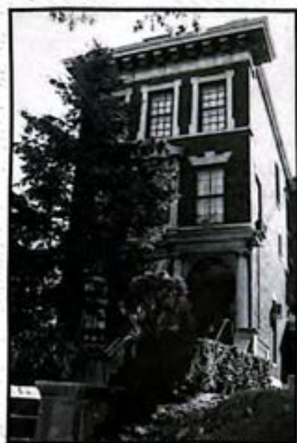
The home of the Rebbe and Rebbetzin on President Street, in Crown Heights.
