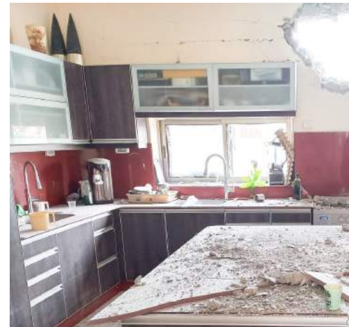
The Pizems' destroyed kitchen.
